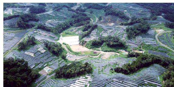
Kanoya Osaki Solar Hills Solar Power Plant
